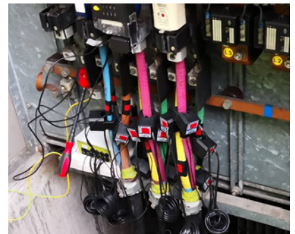
Installation of sensors in the distribution network
