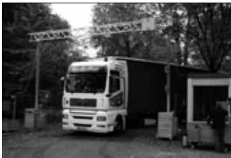
Figure 4: RFID Gate at construction site access road [3]
